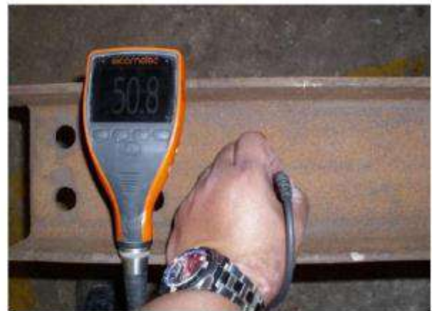
Mill scale with 80% rust ( \text{Fe}_2\text{O}_3 ), thickness is 50.8 microns.
